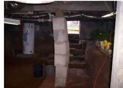
Like getting rid of that stack of concrete blocks and supporting the floor properly. To this end, I have dug a hole ALL the way down to 9 feet below the floor joists in this solid packed clay. Placing the excess dirt along the driveway to bring the yard up to level with my edging boards.
