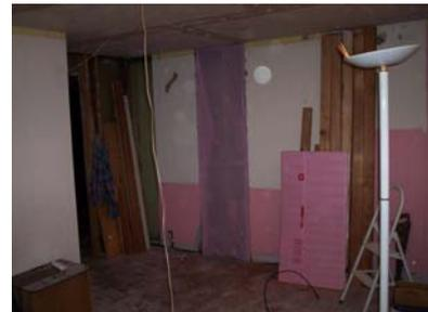
I chose to renovate the ceiling and existing walls and get all the drywall repairs completed before starting on the new closet addition. In the long run it would make the later work so much easier. I also spray painted the windows, mainly to change the aluminum edging to white, but decided to prime and paint the windows themselves also. They would later be painted with the trim paint.
