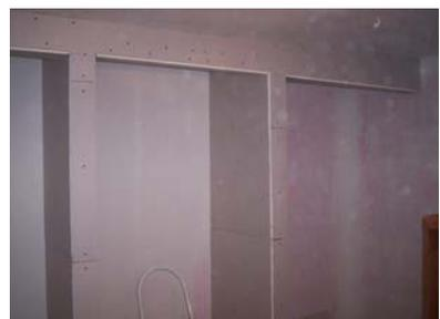
It just dawned on me that NONE of the photos I have shown so far disclosed where the door to the room was. In order to make the closets work out where they are, I had to relocate the existing door 2 inches to the left of where it was originally. It also works out better there too. And of course, I couldn't be working without my FUEL, a can of Pepsi, hi hi.....
