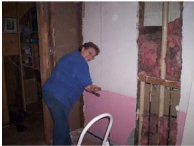
Every contractor NEEDS a GRUNT, so I put Debi to work trimming drywall edges back to the center of studs.
