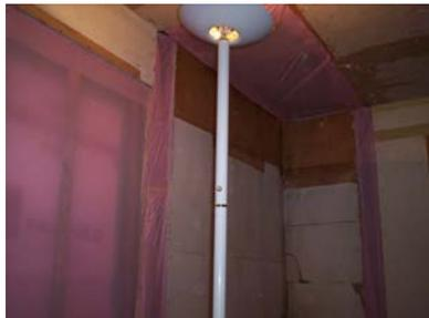
Then I had to insulate and install a vapor barrier along any outside walls. At the same time I decided to install a vapor barrier by the washer/dryer plumbing so that a leak in that area would not damage this room.
