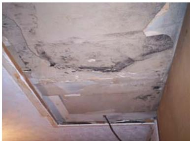
After I began the removal of the original closet, I find that we have two ceilings in this room, separated by 3/4 inch furring strips. The original ceiling severely water damaged. In addition, the original drywall walls inside the closet had never been taped, the upper storage area had never been painted and these walls were also heavily water stained.
