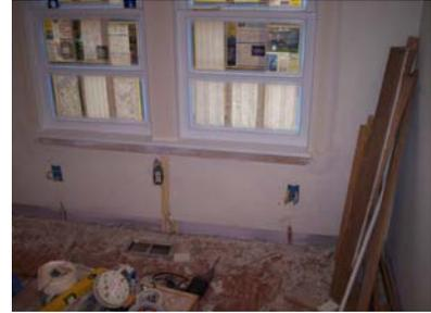
The first photo in this section is the east wall. The outlet on the left is another 4 line phone. The center photo shows the metal ceiling pull box that will hold the ceiling fan. It is wired such that the lighting will be on a dimmer switch and the fan on a separate switch. It is also very heavily braced to hold my own weight when hanging from it. The right photo shows all the preliminary restoration work completed and now ready for priming and painting.
