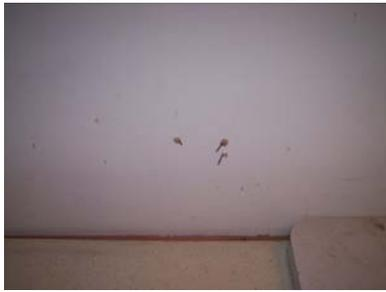
After cleaning off the home built dresser, we find three nails protruding through the wall. These nails are holding the washer/dryer water and waste assembly in the kitchen laundry area, so they just couldn't be cut off.
