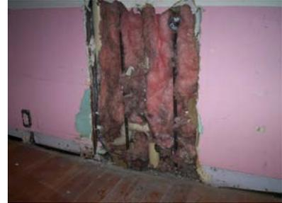
After the home built dresser was removed, we find a severely water damaged wall. This gave us access to the area the nails were protruding from so that a new support could be installed between the studs.
