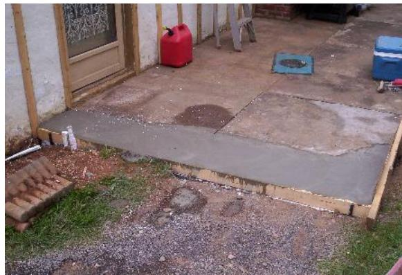
Moving around to the back of the house. We needed to both extend the old patio and add a footing for the walls. Near the wall, you can see the styrofoam used to retain the concrete below ground level, and under the lead edge board as well, just barely.
