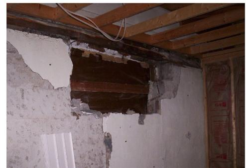
I installed 2x12 in the attic above the floor and across the gable wall, to facilitate removal of the old beam and installation of a new beam with a sheet of steel sandwiched between two 2x10's and capped on the lower side with a 2x6. Afterwards, I could begin removing the remainder of the block wall.
