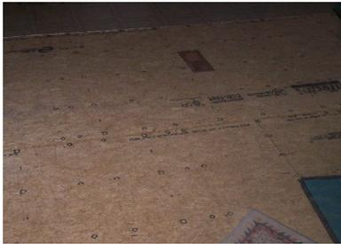
After cutting and removing the flooring we then removed some of the original sub-floor and replaced both layers with new floor sheathing and installed ductwork where it would align with the end of the kitchen base cabinets, it is a breakfast bar with stools.
