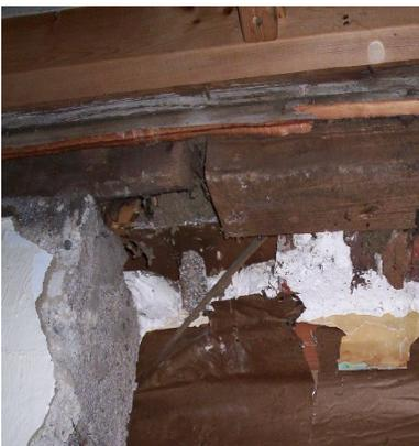
It was looking good until I removed more blocks to find a seam that would require strengthening before any more of the wall could be removed.
